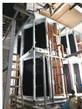
Conducted performance enhancement work of an air-cooled condenser at Regal Hongkong Hotel.
