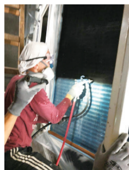
Conducted performance enhancement work of an air-cooled condenser at Regal Hongkong Hotel.
